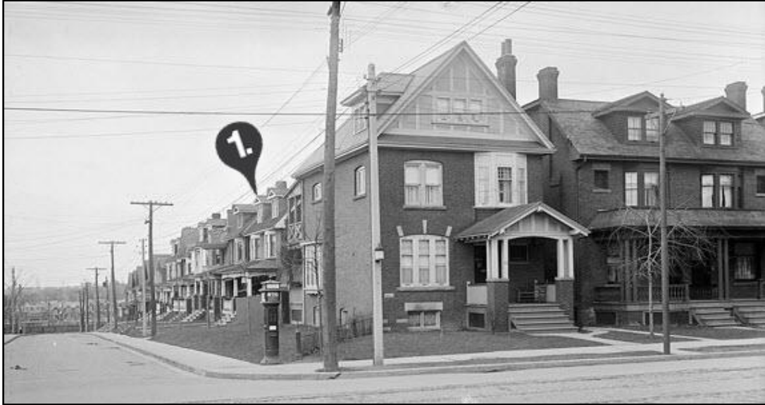
Looking west along Pearson Ave., across Roncesvalles Ave. 1) Tregaskes residence at 206 Pearson. "92 Roncesvalles." 1916. City of Toronto Archives, Series 372, s0372_ss0058_it0545
