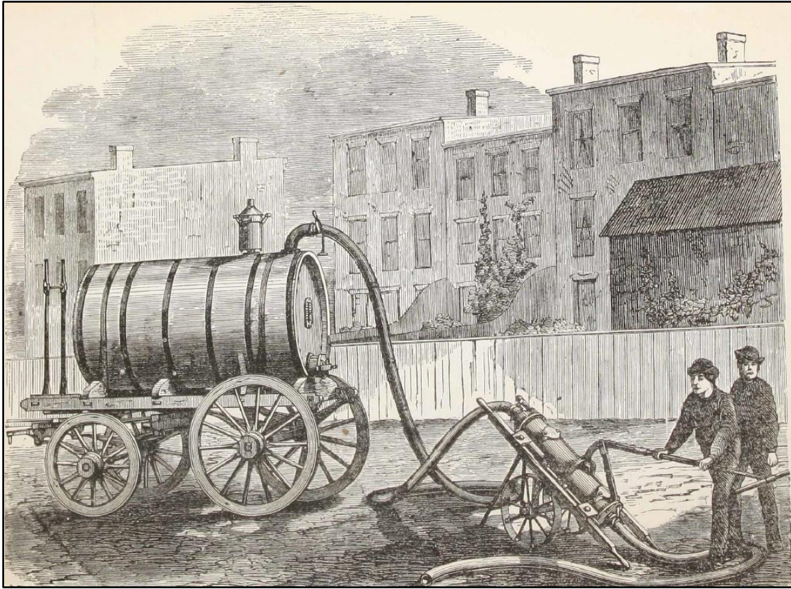
"The odorless excavating apparatus for emptying vaults, sinks, cesspools", by Odorless Excavation Apparatus Co. (Lewis R. Keizer, William Painter). Pub. John Murphy, Baltimore, MA. 1875. Page 8.
